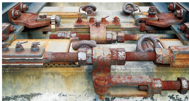
脱落防止座金 Bolt Drop Prevention Washer
