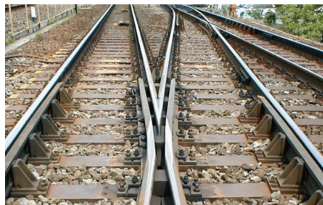
NEWクロッシング NEW (Non-gap Electron beam Welding) Crossing
