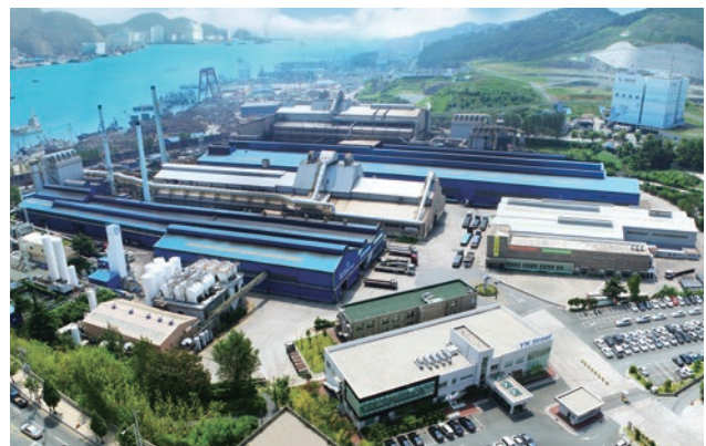
Exterior view of YKS
