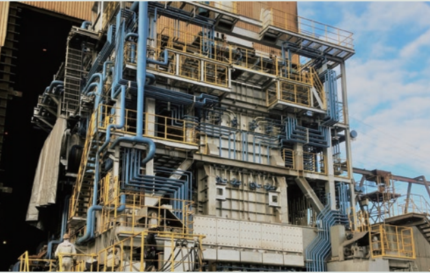
Single-stage furnace top scrap preheater (SSP)
