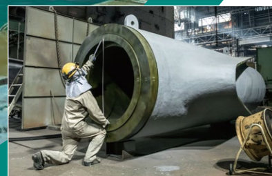
鑄鋼部門 Steel Casting Department
