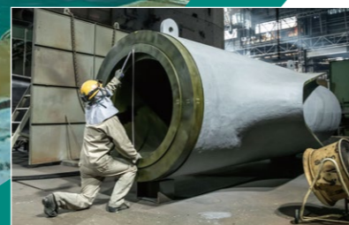
鑄鋼部門 Steel Casting Department
